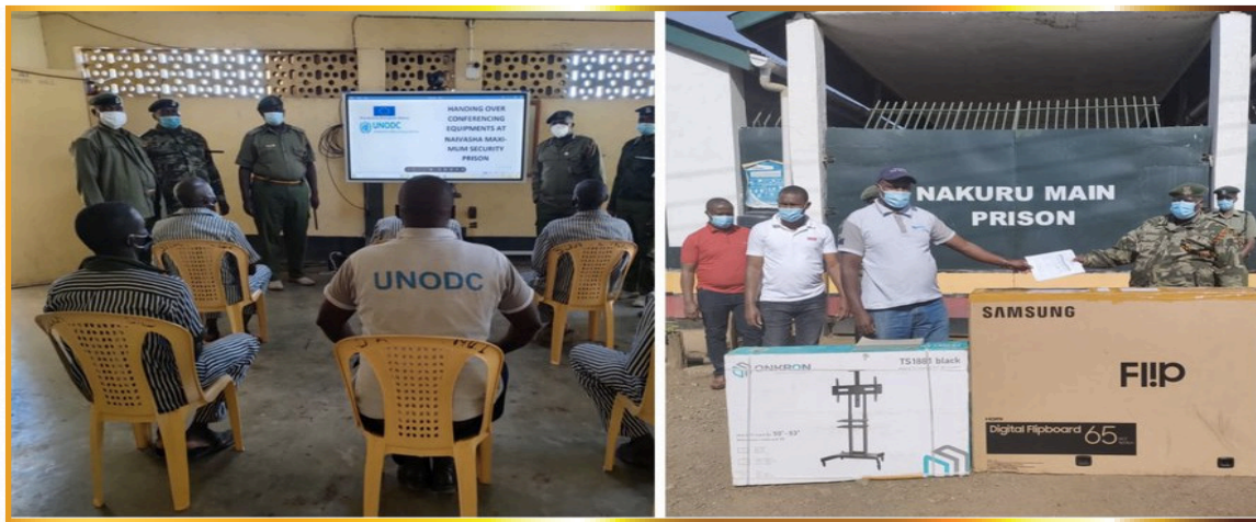
UNODC through EU funded PLEAD Programme installing video conferencing equipment in 12 prisons in Kenya to support virtual hearings.
